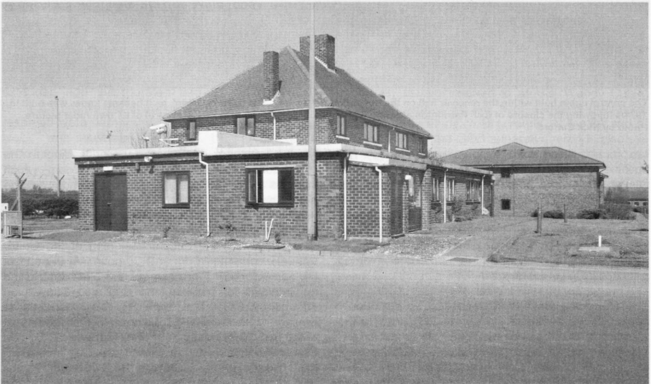
The only building remaining from the Chain Home days is the pair of Air Ministry wardens houses which have now been extended and are used for administration. Photo by Nick Catford
